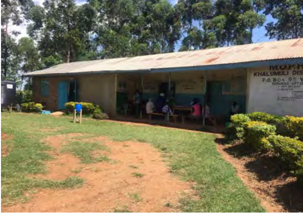
AHAP facility: Khalumuli Dispensary
